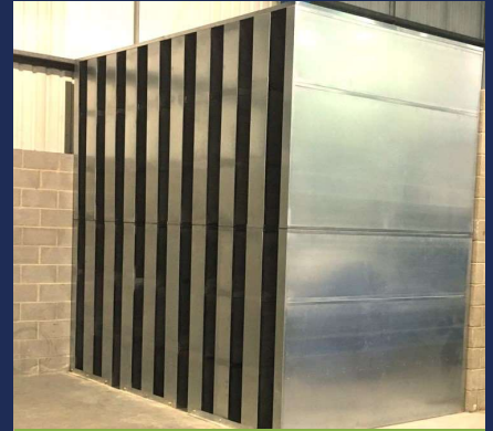
SITE-ASSEMBLED ACOUSTIC BAFFLES
